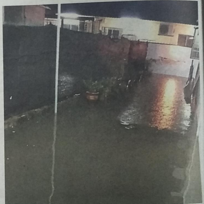
Two bungalows on Jalan Union 1-3 in Sentul get flooded whenever it rains heavily.
