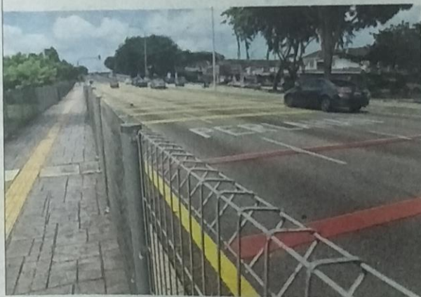
New safety features for the pedestrian crossing in Persiaran Tujuan include speed breakers. — Photos: SAM THAM/The Star
